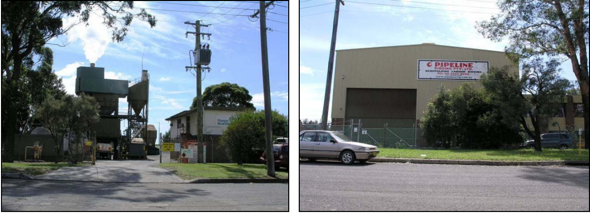
Figure 5 - Photos: Rivulet Crescent, Albion Park Rail
