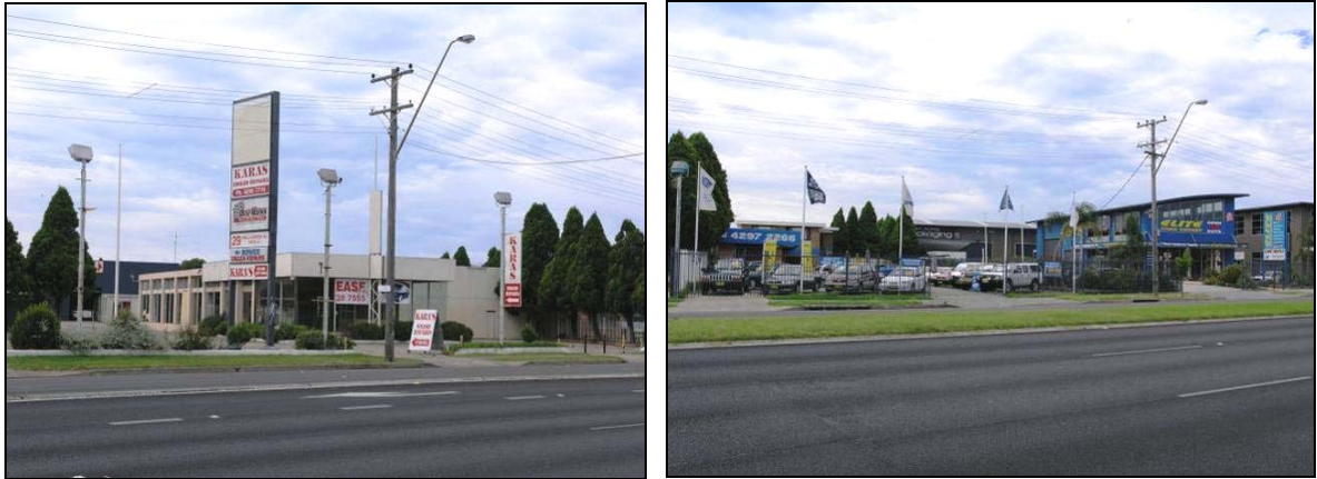
Figure 27 - Photos: Princes Highway, Warilla
