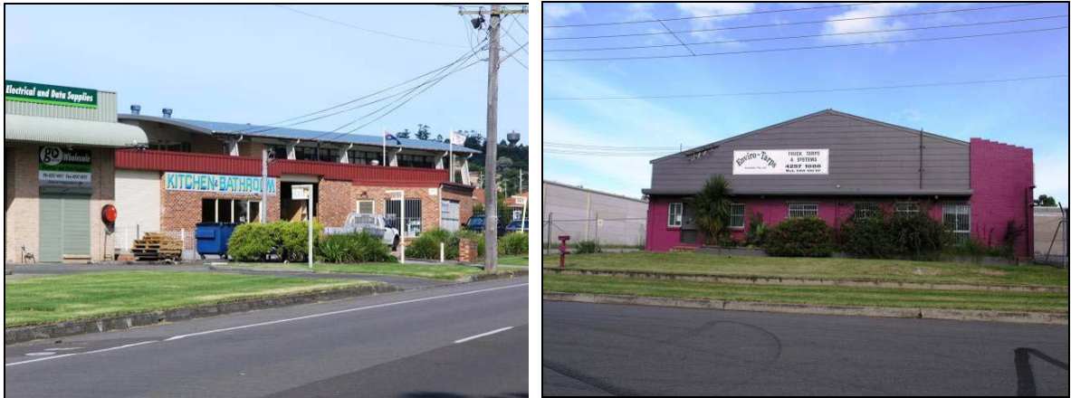
Figure 18 - Photos: Industrial Road, Oak Flats
