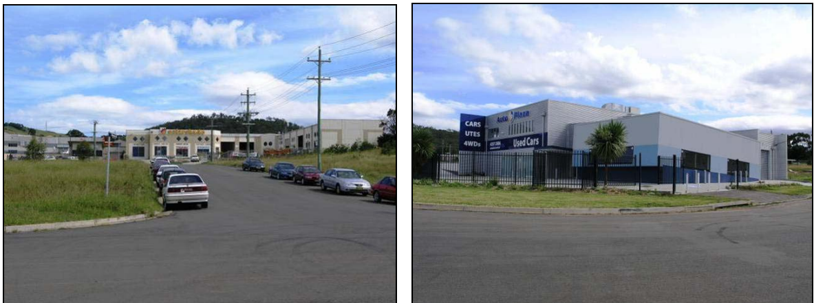
Figure 24 - Photos: Shandan Street, Central Business Park
