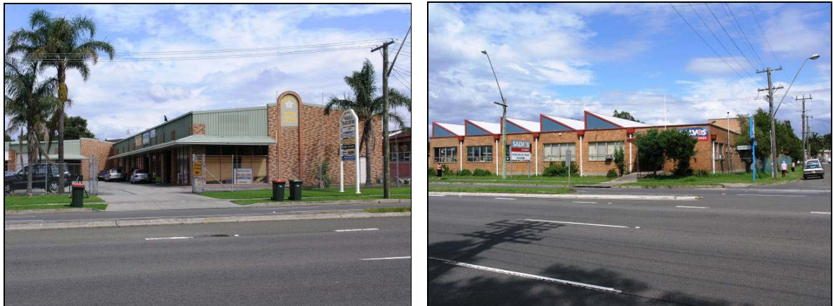
Figure 33 - Photos: Princes Highway, Barrack Heights
