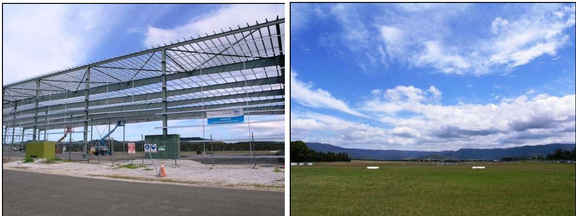
Figure 10 - Photos: Airport Road, Illawarra Regional Airport
