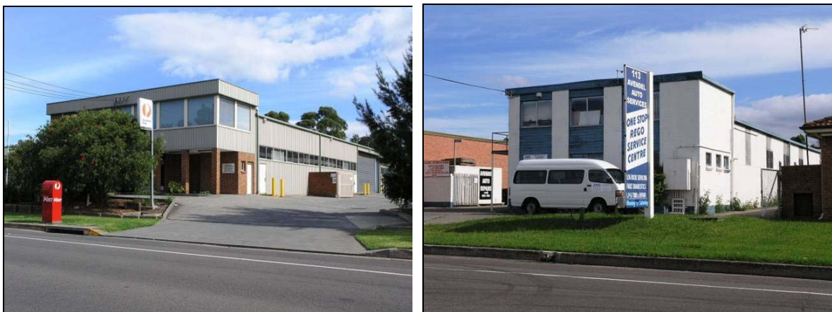
Figure 17 - Photos: Industrial Road, Oak Flats
