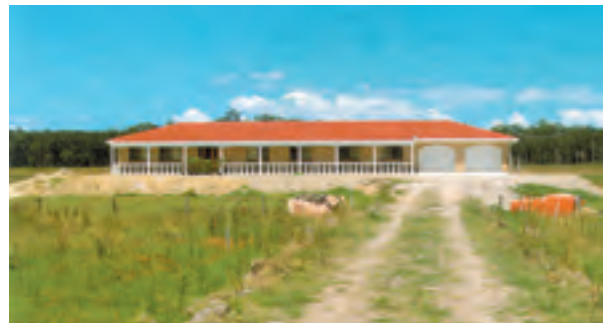
PLATE 12 - Flood Proofing with Fill
