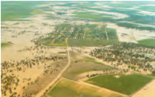
PLATE 13 - Ring Levee Protection
