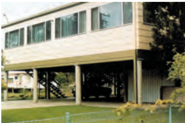
PLATE 9 - Flood Proofed by Raised Floor Level
