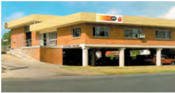
PLATE 11 - Flood Proofing of Commercial Development
