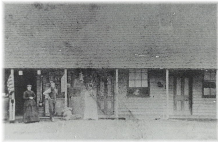
The Settler's Arms Hotel, Shellharbour, c.1865. (Shellharbour Images, SCC).
