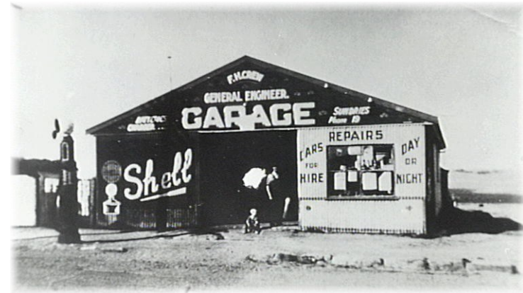
Shell Garage, Shellharbour, 1926, built by Ted Thomas and leased by Frank Crew and later by his brother Alf. (Shellharbour Images, SCC).
